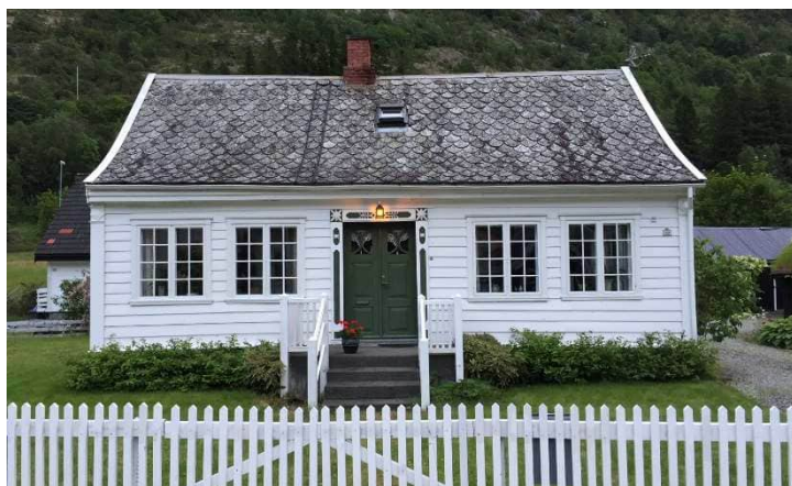
Figure 4 - House in Lærdalsøyri with about 10% glazing to the front wall (including projected area of roof)
