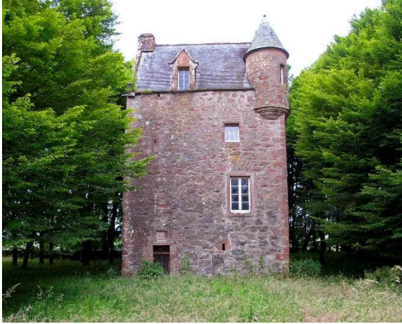
Figure 5 - Fourmerkland Tower (Scotland) with about 4% glazing to the front wall (Picture by Arjayempee on Flickr)
