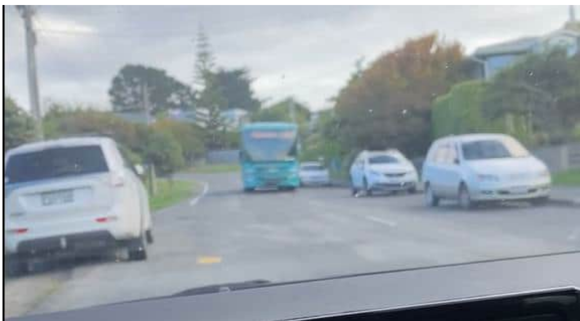
Image 1: With cars parked both sides, even with the car on the left pulled ½ off the road, there is insufficient room for a car and bus to pass on this relatively straight section of road
