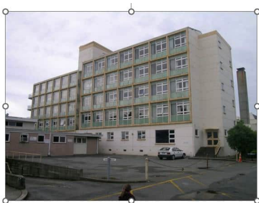
Nurses' Hostel on former Women's Hospital site (five storeys), prior to demolition in 2009
