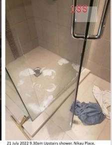
21 July 2022 9.30am Upstairs shower. Nikau Place, unable to drain away due insufficient waste water network capacity/overflow from stormwater network. If we had flushed the toilet the bowl would likely have overflowed.
