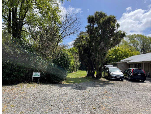
Photo 2: View of rear of Tea House building looking west
