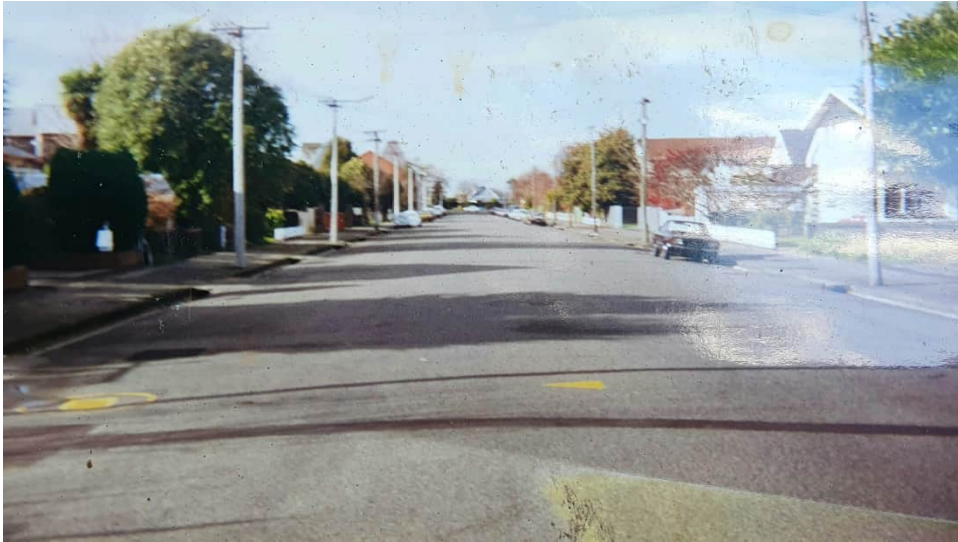
The Eastern half of Chester Street East prior to CCC development in the 1980's
