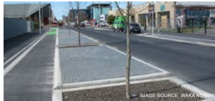
IMAGE SOURCE: WAKA KOTAHU CUMBERLAND STREET
