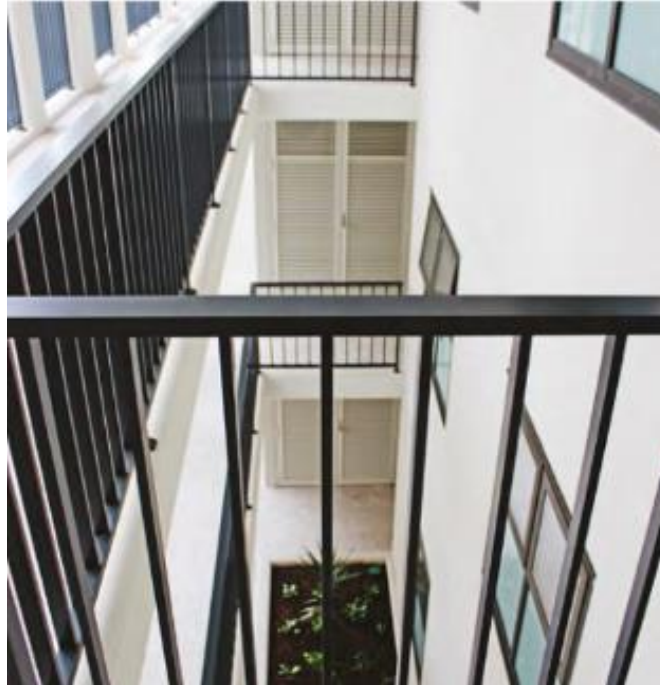
Figure 30: Open gallery access is separated from apartments to allow for glazing and privacy (Source: WAPC, 2019)
