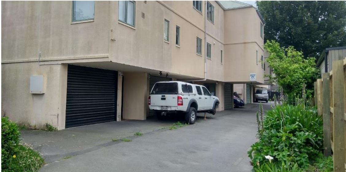
Figure 31: Vehicle access and parking dominates the ground floor, with overhangs creating CPTED issues due to a lack of overlooking and creation of entrapment spaces. There is a lack of stewardship of the space as a result.
