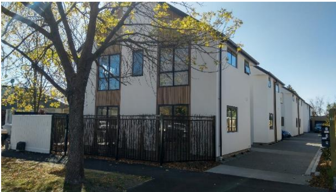
Figure 33: An example of moderate to high (50%) site coverage.
