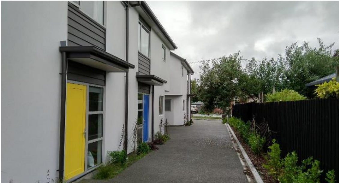
Figure 26: Ground floor living with garaging consolidated in between units minimises the visual and experiential impact of on site carparking.
