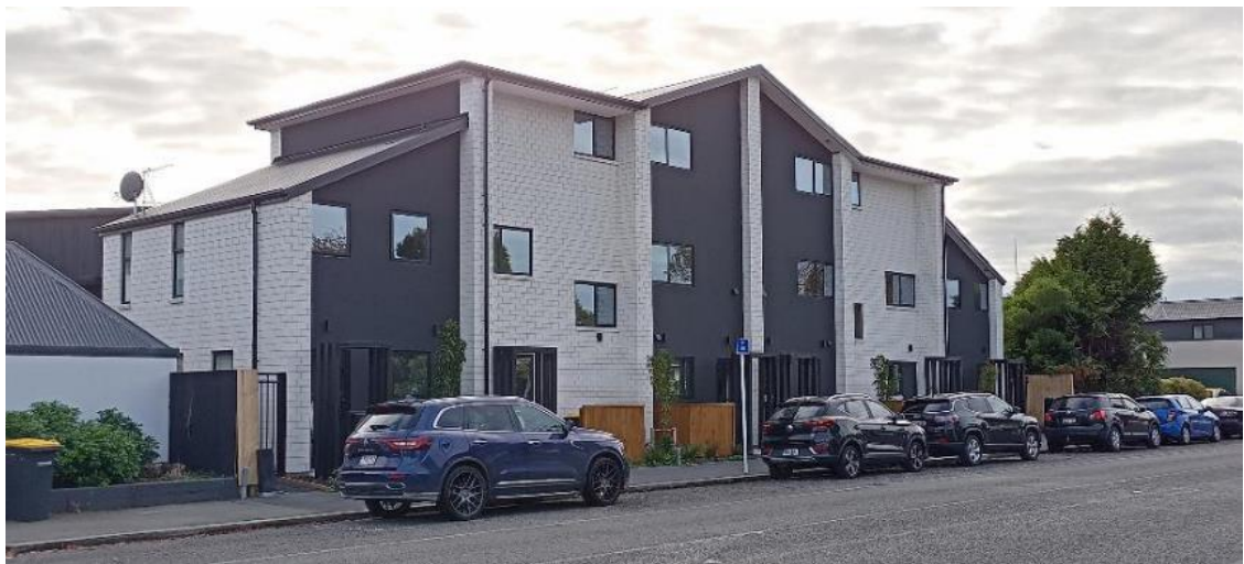
Figure 13: Sections of the building adjacent to the boundaries have been shaped by the recession plane angles to maximise buildable area.
