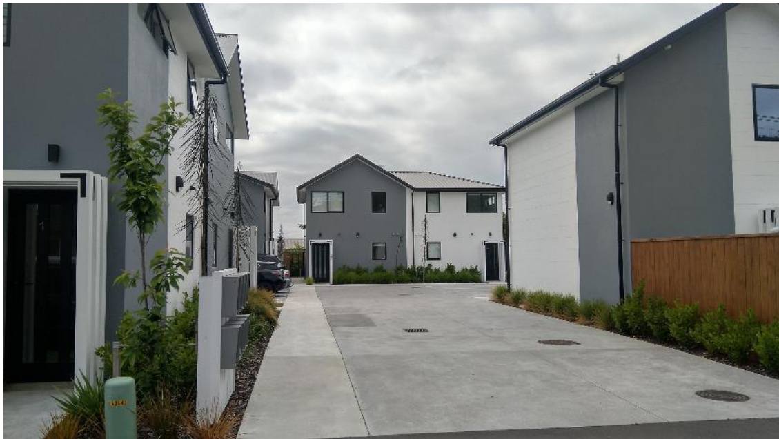
Figure 23: This driveway from a collector road to 8 units has adjacent planting but is wide, with the pedestrian access at the same grade (un-dedicated) making it appear wider and providing the opportunity for parking over pedestrian access.
