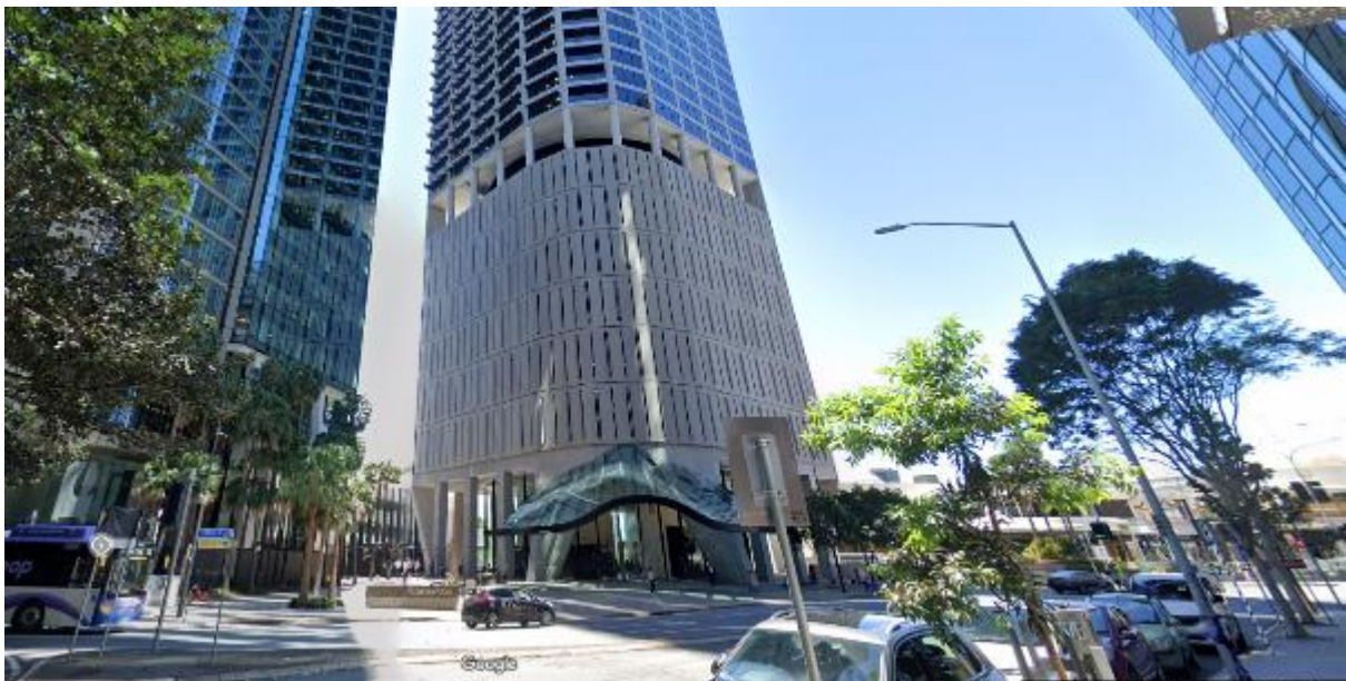
Figure 13: Riparian Plaza, Brisbane. Lower levels are utilised for car parking reduces the extent of engagement from street level experienced in respect to the building adjacent.
