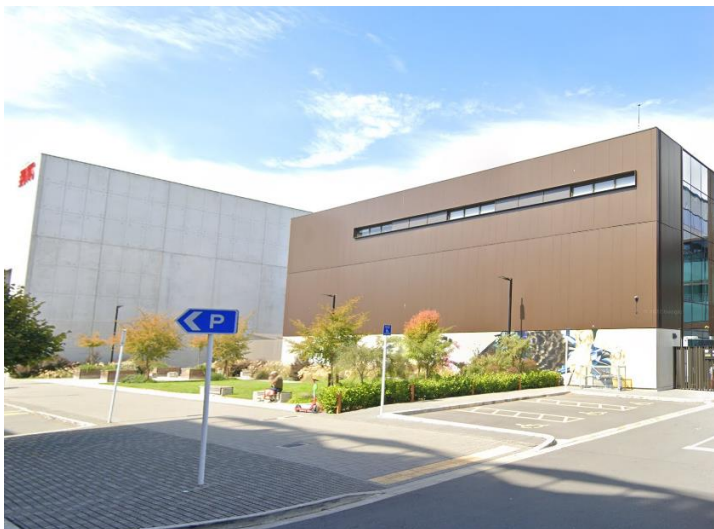
Figure 10: Flank walls with varying facade treatment in Ōtautahi Christchurch.
