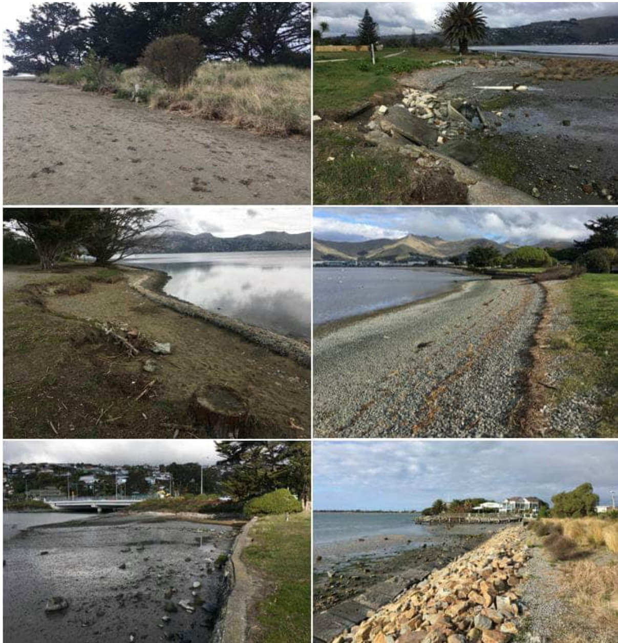
Figure 4.27: Site photos (taken August 2020) around the Avon-Heathcote estuary shoreline. (Top left) natural unconsolidated shoreline on the western side of Southshore spit (Cell 15), (top right) rip rap along the unconsolidated shoreline near Penguin Street (Cell 17), (centre left) eroded shoreline near South New Brighton Park (Cell 19), (centre right) gravel shoreline near Windsurfer's Reserve (cell 24), (bottom left) protected bank near Humphreys Drive (Cell 25), (bottom right) protected bank near Beachville Road (Cell 26).
