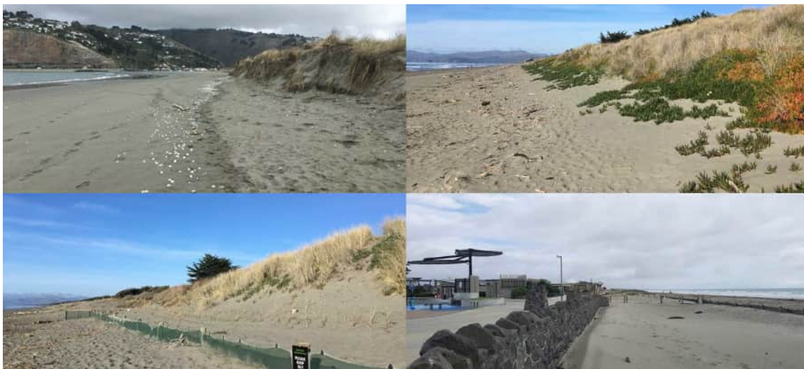
Figure 4.1: Site photos along Christchurch open coast. (Top left) Erosion scarp on Southshore Spit, (top right) vegetated, accreting dunes near Waimairi, (bottom left) dune planting and fencing near Waimairi, (bottom right) seawall at New Brighton.
