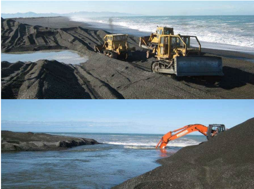
Figure 2.16: Bulldozers removing the 'scab' to make the connection between the cut and sea (top). Excavator working to enlarge the freshly open cut (sourced from Measures et al., 2014)
