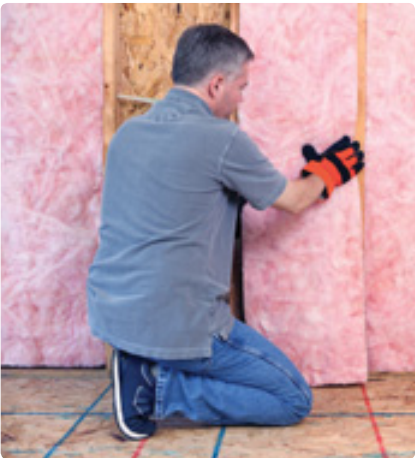
Left: Insulation installed during construction helps make a building more energy efficient.
