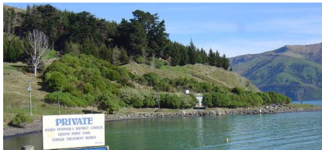
Akaroa Waste Water Treatment Plant: Greens Point
