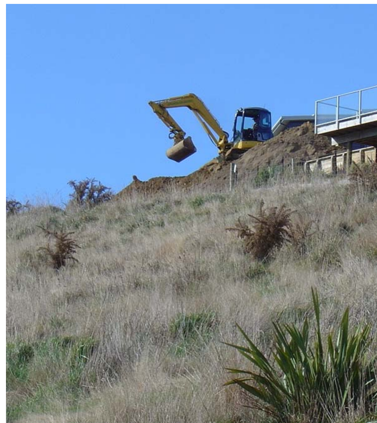
Changing land use and development - land being developed at Ngaio Point as part of a new subdivision.
