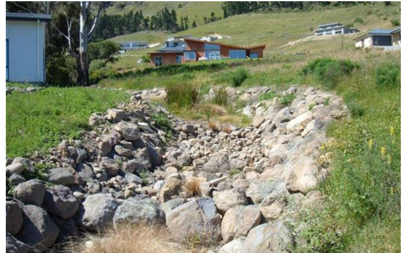
An example of a constructed, naturalised stormwater drain from a low density development on the Port Hills (Photo courtesy of Christine Heremaia)
