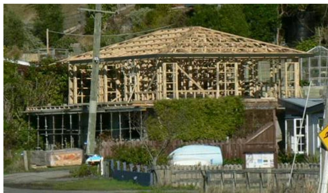
New house being built in Wainui
