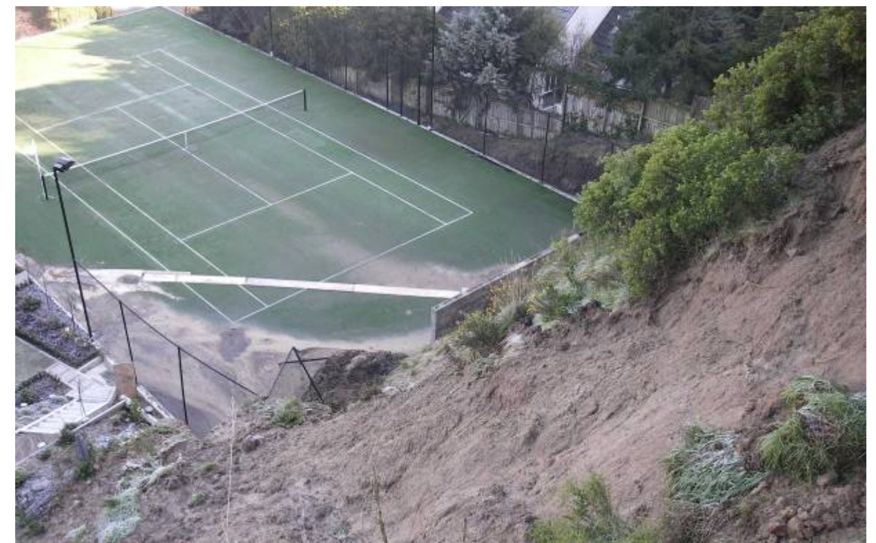
An example of slope instability and landslide on Huntsbury Hill, Christchurch Urban Area (Photo courtesy of Barry McDowell)
