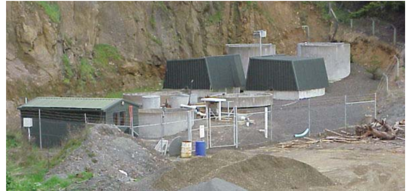
Duvauchelle WWTP, located in an old quarry beside State Highway 75, between Pawsons Valley Road and Pipers Valley Road (Photo source: BPDC Activity Management Plan)
