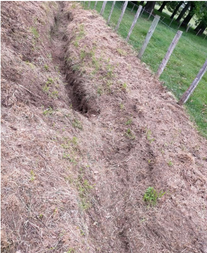
Area cleared with weed eaters by CCC but still clearly seriously blocked.
