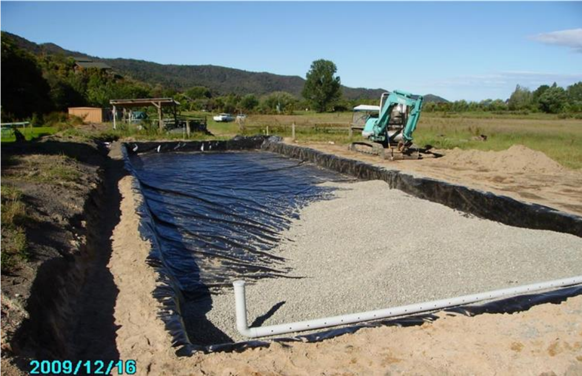
Figure 4.7 – Construction of a Subsurface Flow Wetland (at Abel Tasman courtesy of Cameron Gibson and Wells Ltd)
