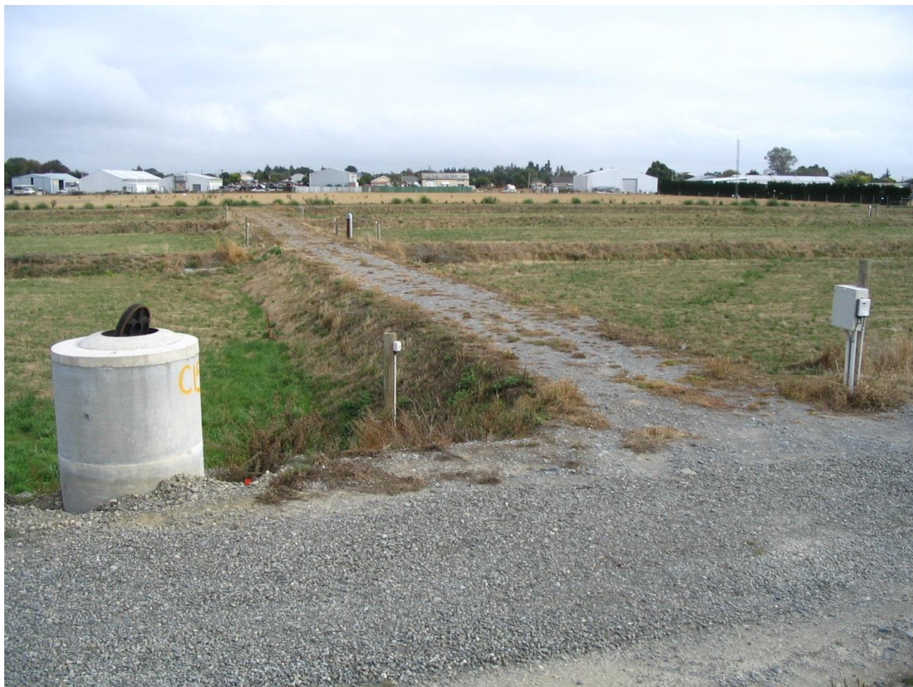
Figure 4.12 – Infiltration Basins at Leeston
