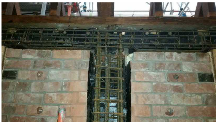
Installation of the reinforcing to the Buttress columns and the perimeter ring beam.
