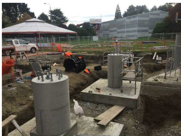
New foundations for the indoor hydroslide
