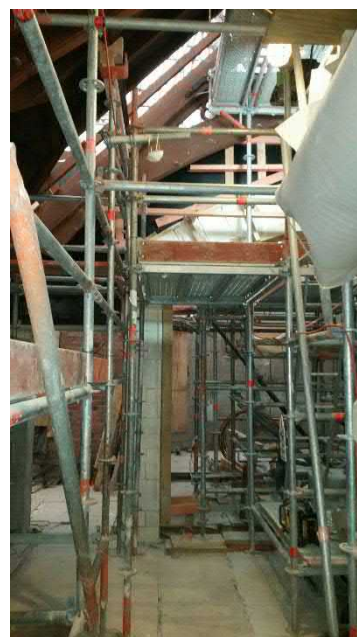
Chancel arch ready to receive the second pour of concrete.
