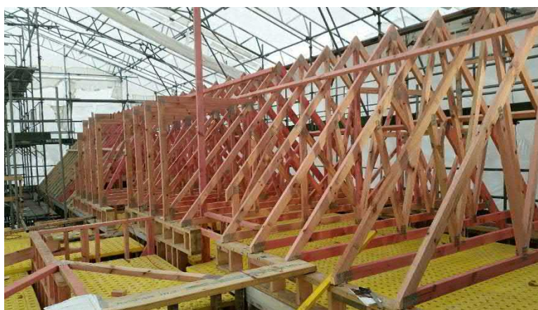
New Trusses being install
