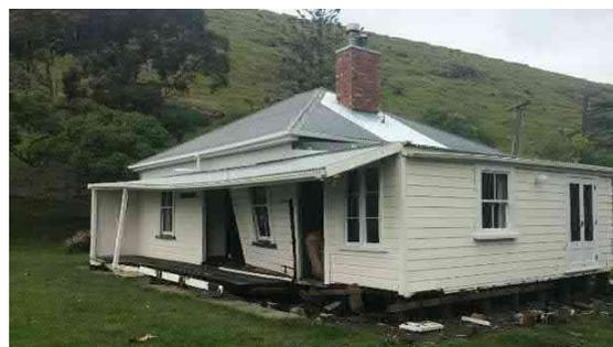
A waterfront cottage in Little Pigeon Bay was damaged and washed off its piles in a tsunami in 2016.
