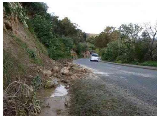
Discharges of storm water from roads is observed damaging banks on both sides of roads.
