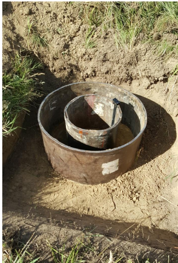
Photograph 9: Infiltration Test IT111 sub-surface within the 'less preferred area' (Site 111).
