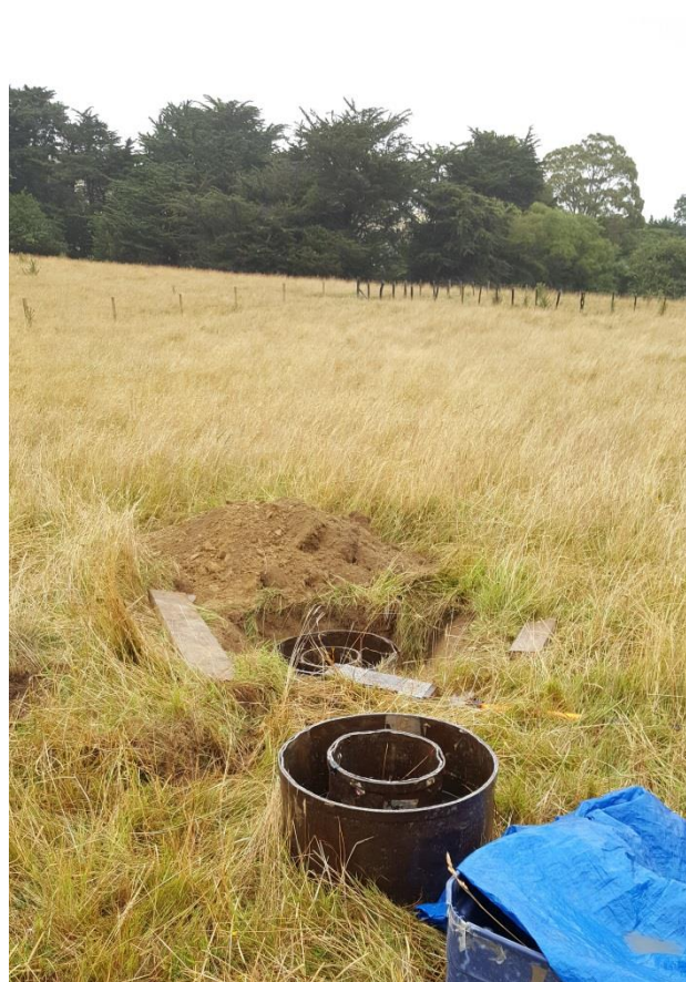
Photograph 7: Infiltration Test IT109 surface and subsurface within Robinsons Bay (Site 109).
