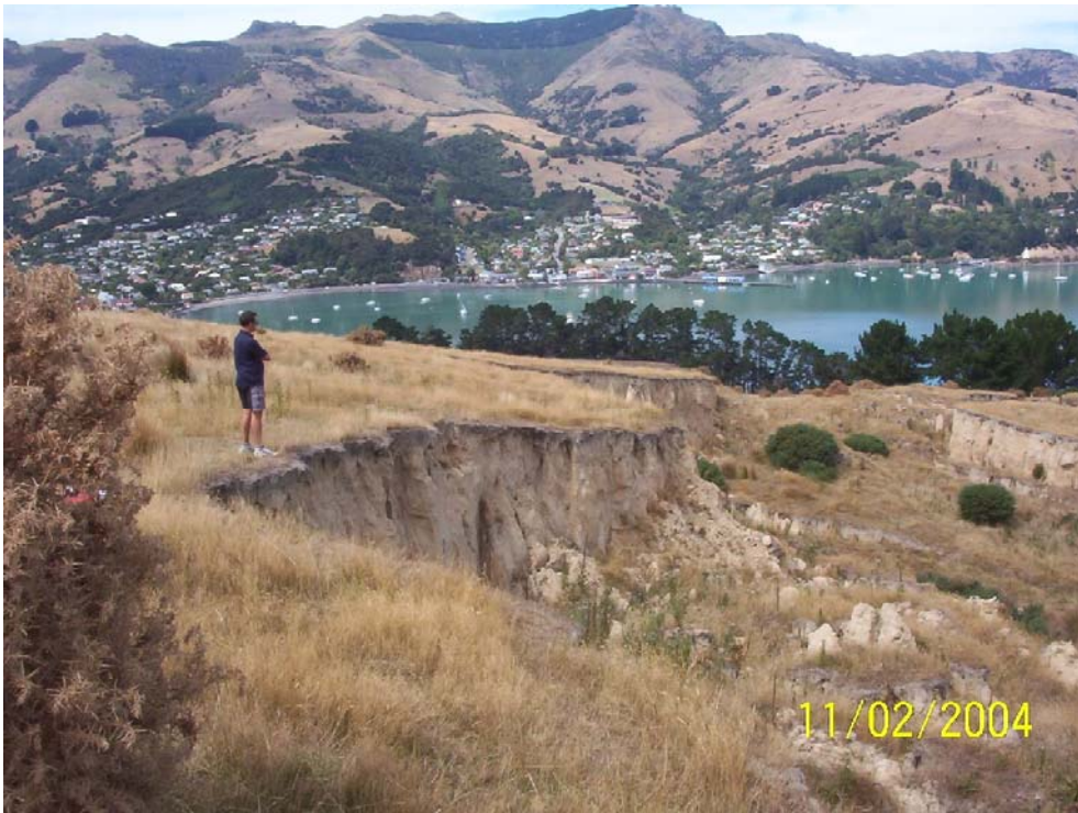
Photograph 1: The head scarp of the western landslide at the margins of the ancient landslide feature that dominates the south facing slopes above Childrens Bav (photograph summer 2004).
