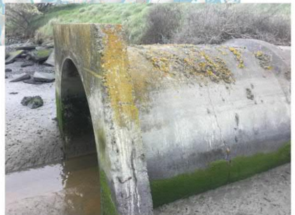
Stormwater pipe outlet on Estuary Drain
