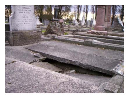
**Example** – concrete slab/vault distortion or collapse, due to compaction of grave fill and/or vandalism
