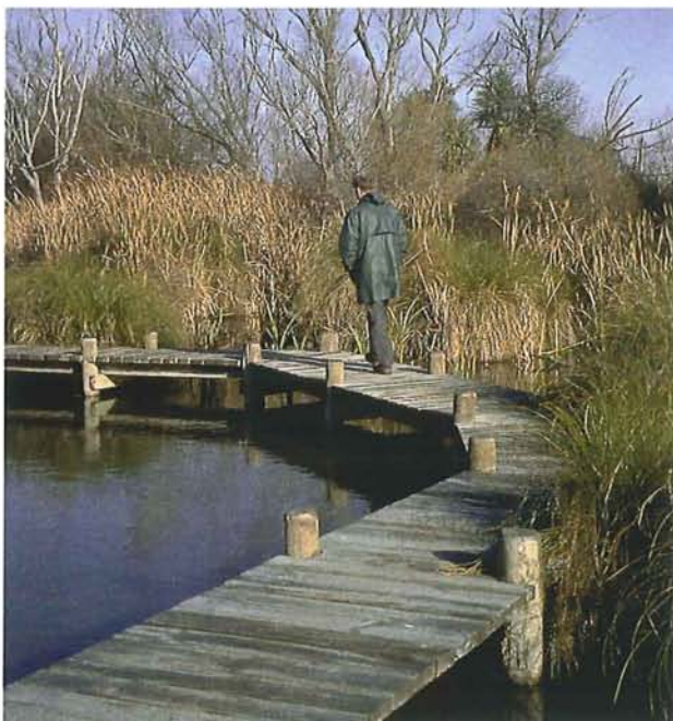
Figure 16-4: Raised walkways provide the public with safe access to a once inaccessible area. However, first consider retaining the area's inaccessibility to facilitate a wildlife refuge area. Ōtūkaikino wetland.
