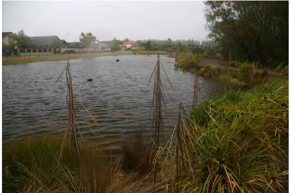
*First Flush Pond at Redwood Springs Designed to Trap Sediment*
