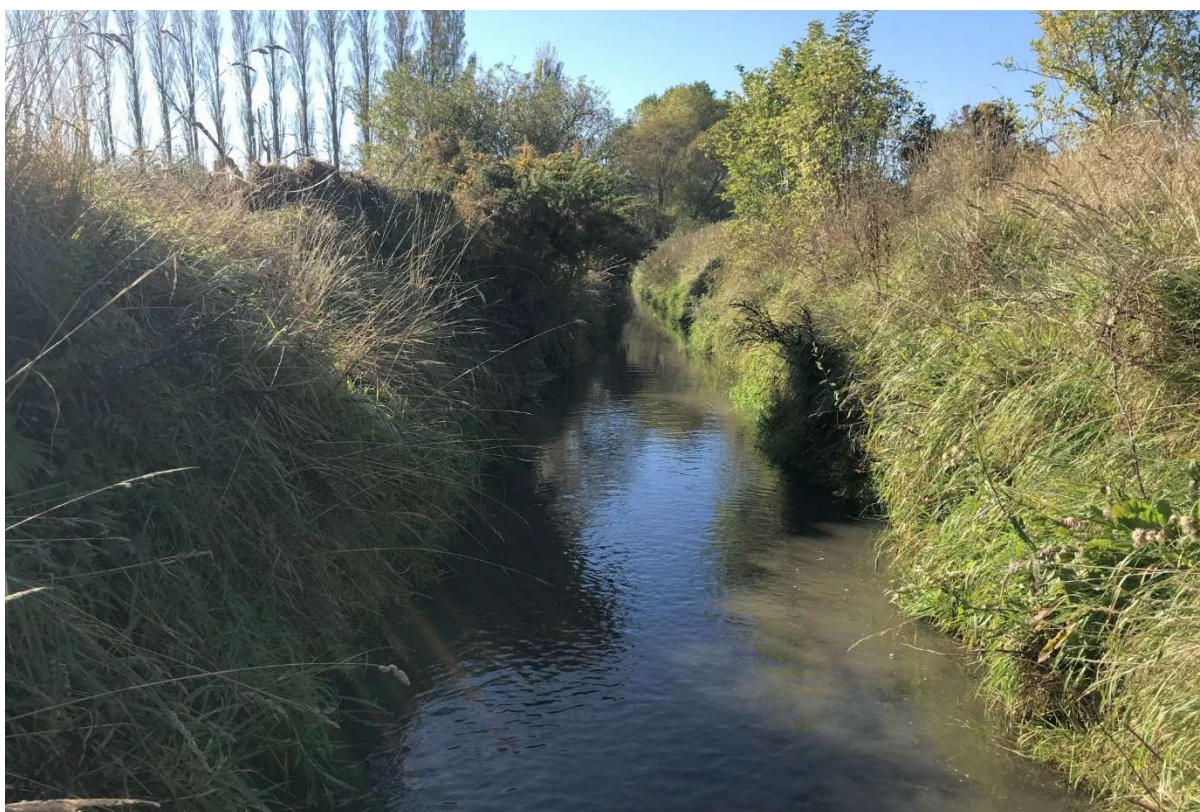
Figure 2: Site B – upstream looking downstream.
