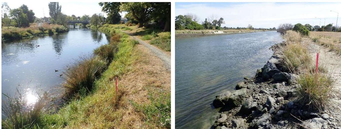
Figure 4: Images from Site 30 at Gayhurst Road (left) and Site 32 at Pages Road (right) illustrate how the lower Avon River is lined by stopbanks, which prevent development of a natural floodplain and associated ecosystems.
