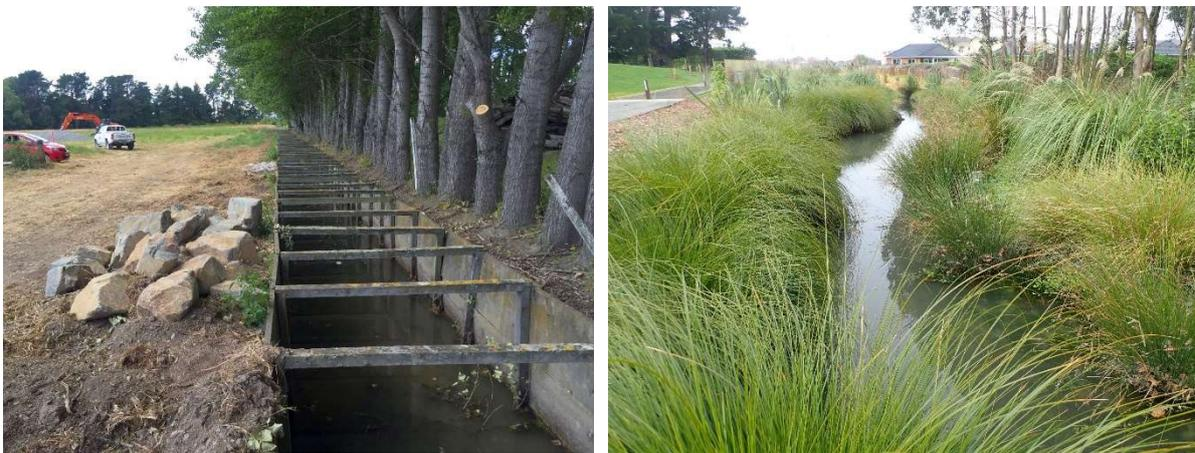
Figure 30: Buller Stream on January 2017 (left) and on May 2019, after waterway restoration (right).
