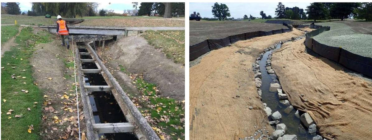
Figure 31: No. 1 Drain in Shirley Golf Course, on May 2017 (left) and nearing completion of restoration work on November 2018 (right).
