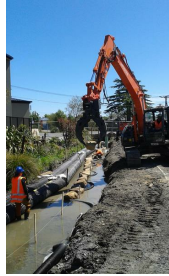
Placing boulders in the creek bed
