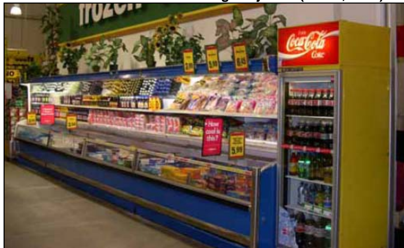
Typical open cover remote chiller cabinets used for holding frozen food, with self-contained drinks fridge adjacent (EECA, 2003)
