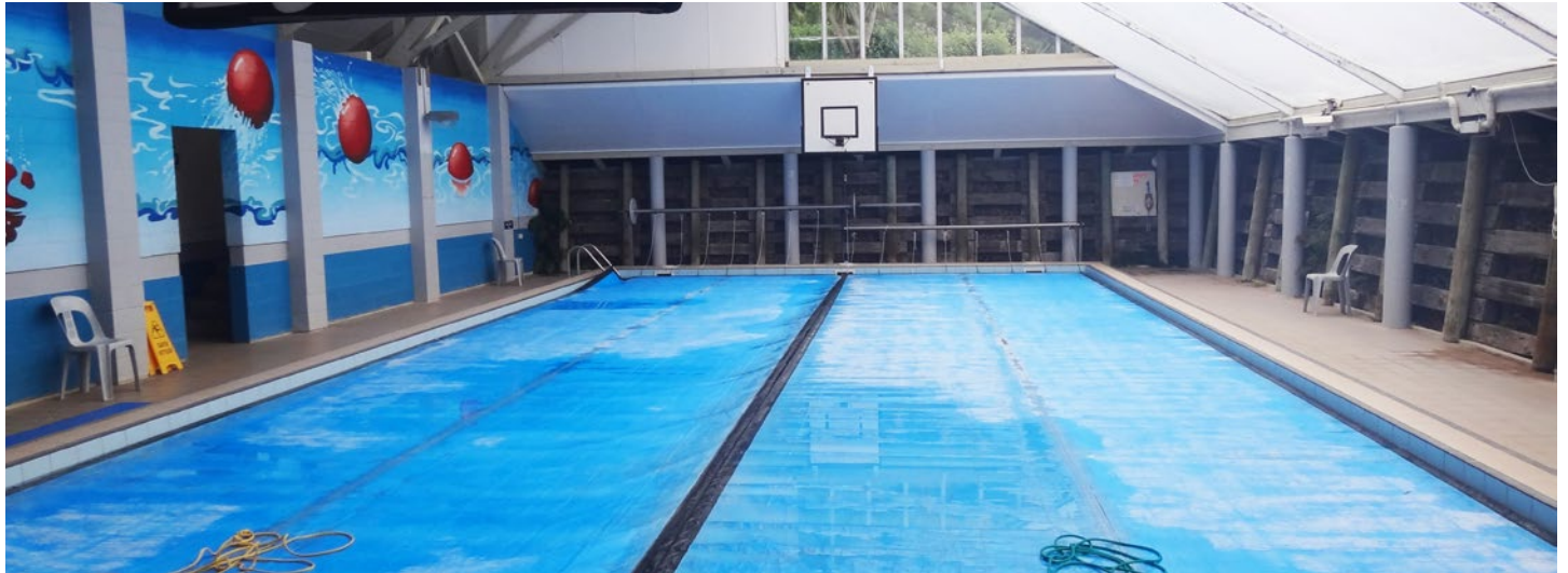
Pool cover to reduce convective heat loss © Copyright
