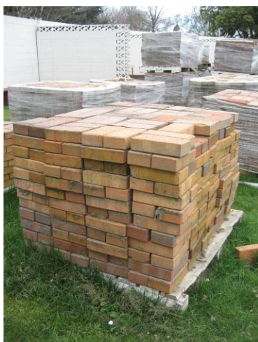
Pavers removed during demolition and re-laid during construction © Copyright
