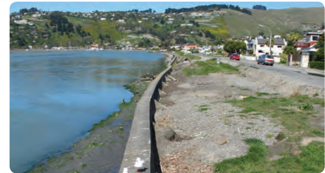
Figure 3.20 - The existing Beachville Rd seawall and space adjacent (Sept, 2012).
