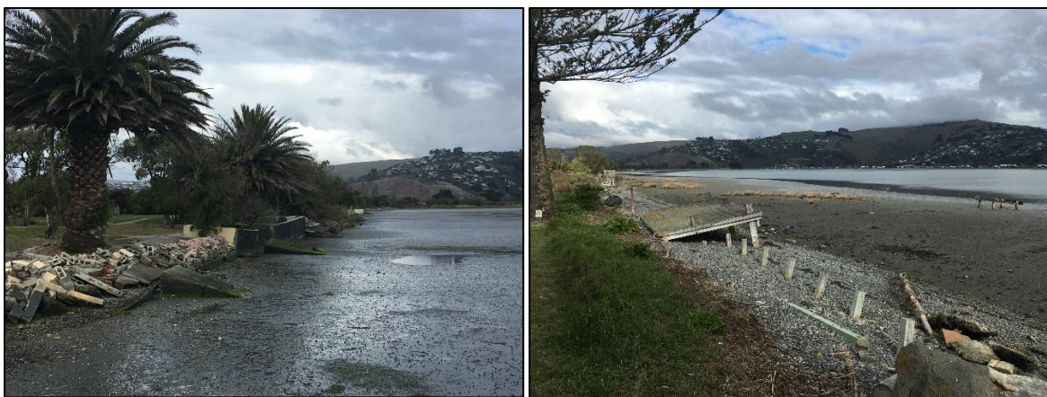
Figure 3.4: Example of informal, non-consented structures along the Avon-Heathcote Estuary
