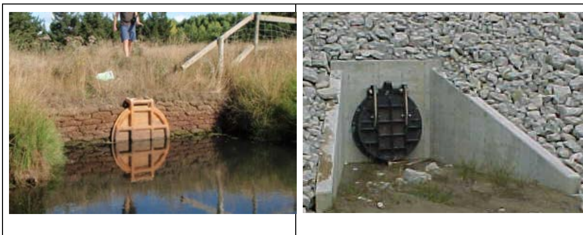
Figure 4-16 Flap gate examples
