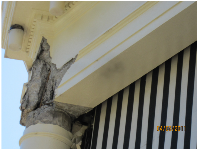
Typical damage and failure of the column capital and dome collar joint with exposed reinforcing steel. The decorative plaster moulding to the capital has collapsed.
