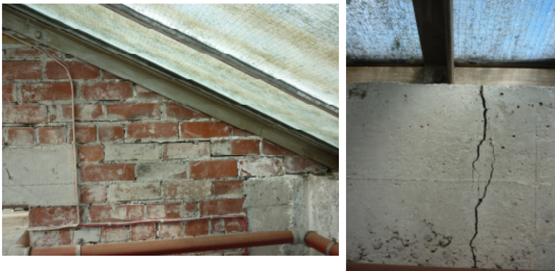
Figure 4-5: (a) Stepped mortar cracking in the skylight bulkheads (b) cracks in the encasing concrete of the skylight steel beams
