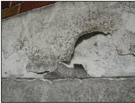
Plaster failure, east elevation (above left) and the movement between capping stones (above right) (DPAL).
