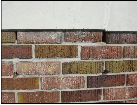
Crack in stringcourse with evidence of loss of mortar in brickwork. (DPAL)
