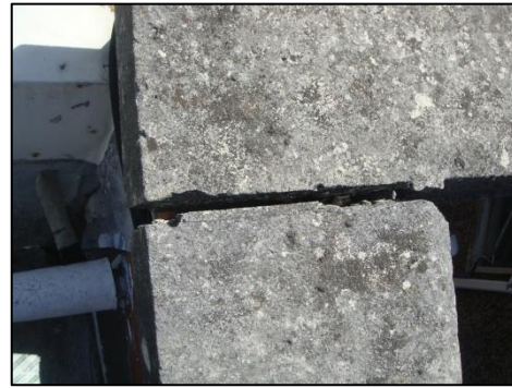
Plaster failure, east elevation (above left) and the movement between capping stones (above right) (DPAL).
