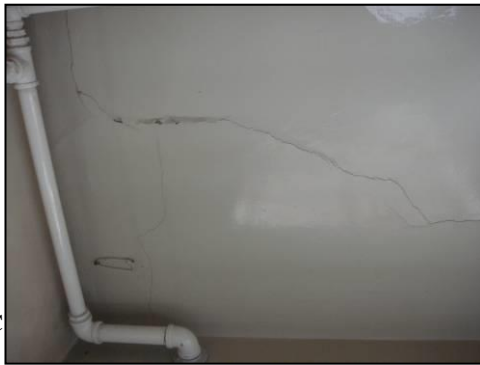
Crack and paint lifting in the wall of the upstairs servery.
