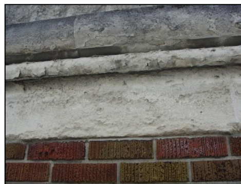
Erosion of stonework. Dirt in the pores reduces the ability of the stone to breathe while the deterioration continues below the outer surface (DPAL).
