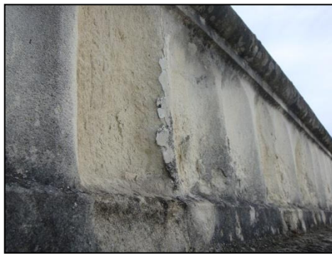
Erosion of stonework. Dirt in the pores reduces the ability of the stone to breathe while the deterioration continues below the outer surface (DPAL).
