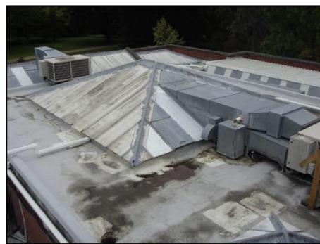
Evidence of water pooling and patched surface
