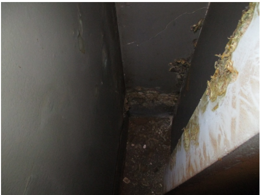
OLD MUNICIPAL CHAMBERS Innovac Room (Ground Floor) Walls. Detail 1 Dry rot in north west corner of room
