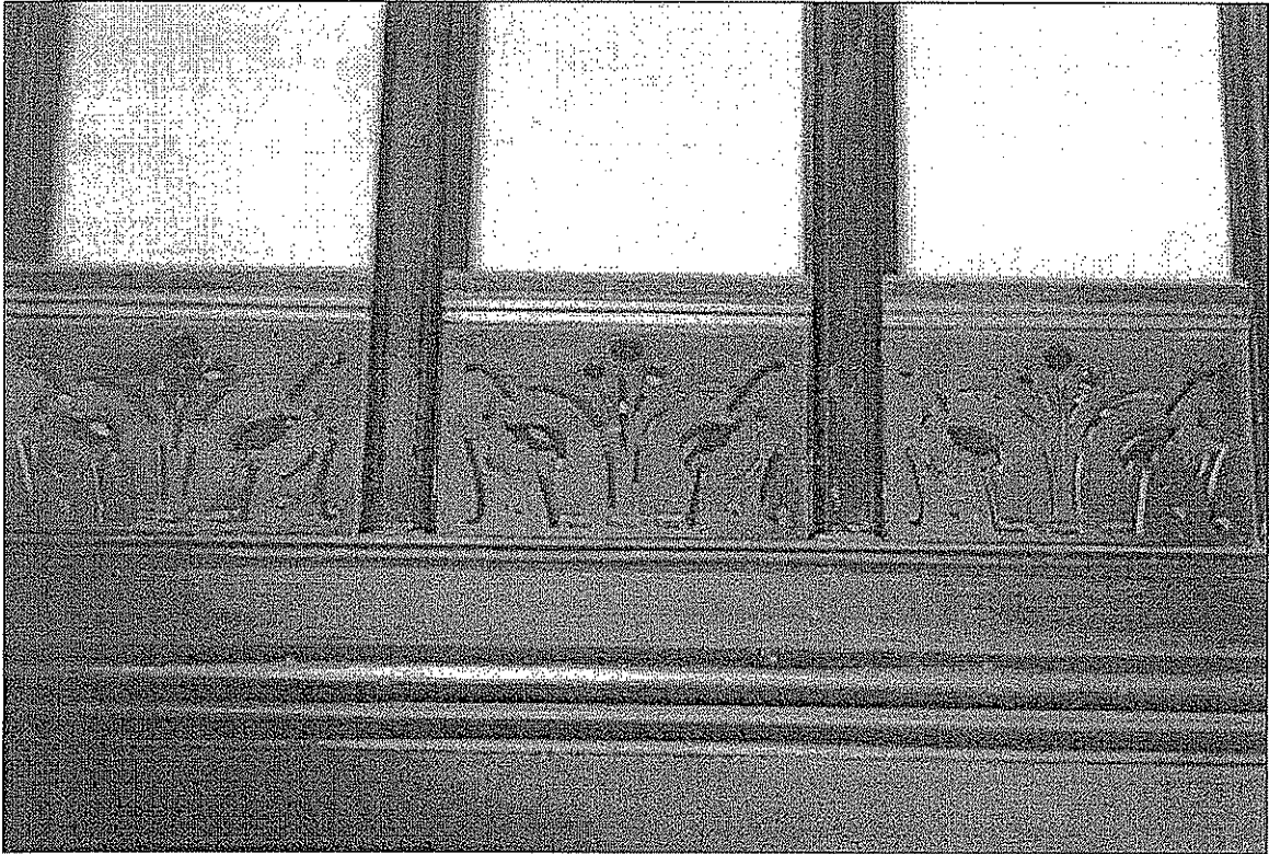
Figure 20: Carved panels in staircase
