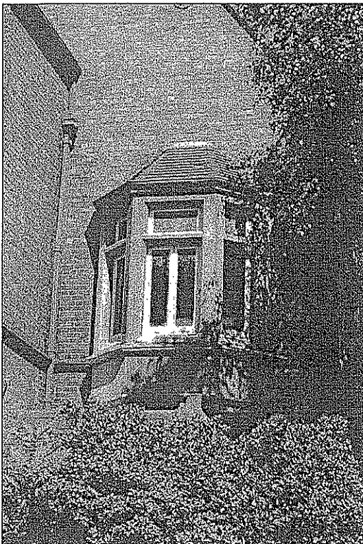
Figure 17: Oriel window on north elevation
