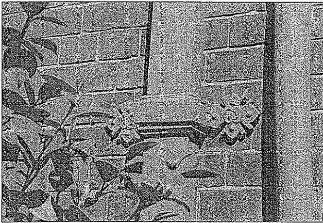
Figure 18: Cast iron downpipes and brackets
