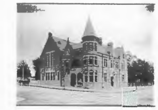
OLD MUNICIPAL CHAMBERS Repairs, Reconstruction & Restoration
