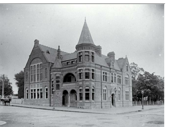
OLD MUNICIPAL CHAMBERS Repairs, Reconstruction & Restoration
