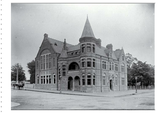
OLD MUNICIPAL CHAMBERS Repairs, Reconstruction & Restoration
