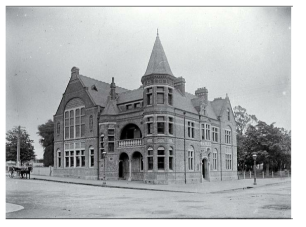
OLD MUNICIPAL CHAMBERS Repairs, Reconstruction & Restoration
