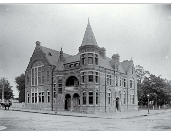
OLD MUNICIPAL CHAMBERS Repairs, Reconstruction & Restoration
