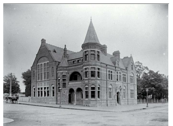
OLD MUNICIPAL CHAMBERS Repairs, Reconstruction & Restoration
