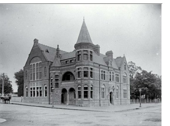
OLD MUNICIPAL CHAMBERS Repairs, Reconstruction & Restoration
