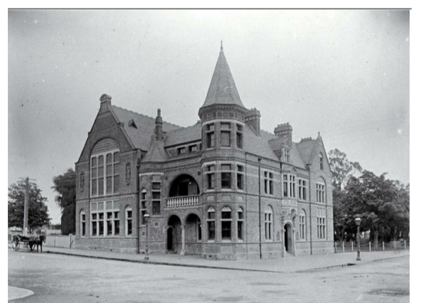
OLD MUNICIPAL CHAMBERS Repairs, Reconstruction & Restoration
