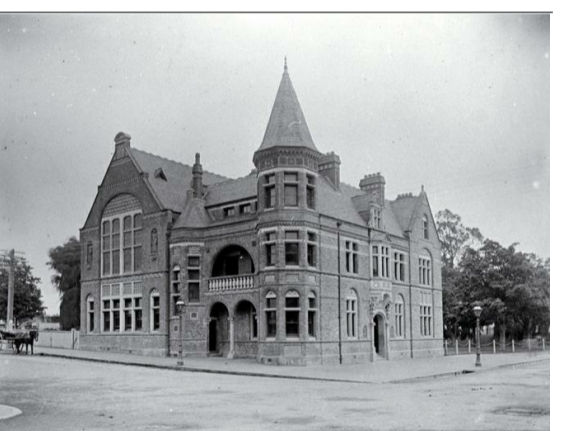
OLD MUNICIPAL CHAMBERS Repairs, Reconstruction & Restoration
