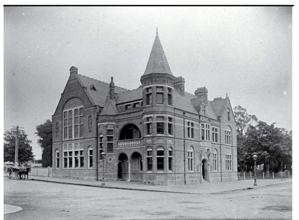
OLD MUNICIPAL CHAMBERS Repairs, Reconstruction & Restoration
