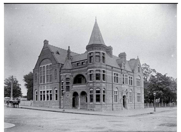
OLD MUNICIPAL CHAMBERS Repairs, Reconstruction & Restoration
