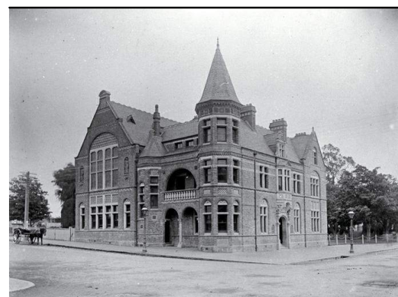
OLD MUNICIPAL CHAMBERS Repairs, Reconstruction & Restoration
