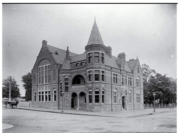
OLD MUNICIPAL CHAMBERS Repairs, Reconstruction & Restoration
