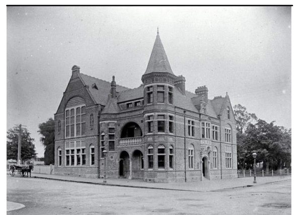
OLD MUNICIPAL CHAMBERS Repairs, Reconstruction & Restoration
