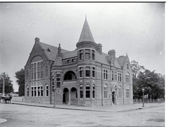
OLD MUNICIPAL CHAMBERS Repairs, Reconstruction & Restoration
