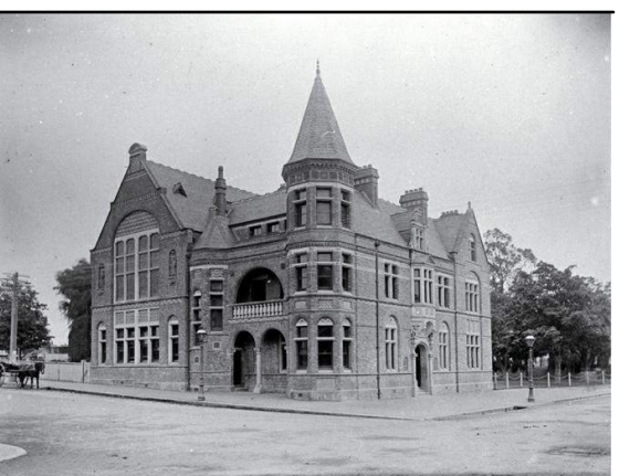
OLD MUNICIPAL CHAMBERS Repairs, Reconstruction & Restoration
