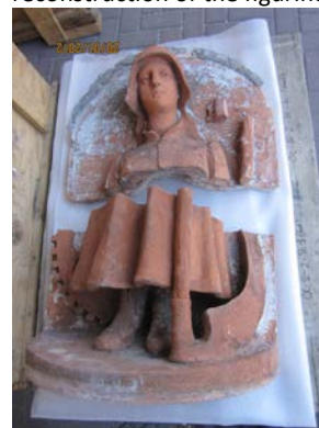
The Figurine, 'Industry', prior to removal showing the displacement of the brickwork securing the panels in place, and after removal. The damaged profiled bricks forming the alcove opening have been recorded and stored enabling the reconstruction of the figurines.
