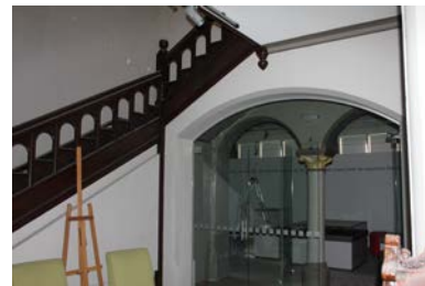
The ground floor stairwell.
