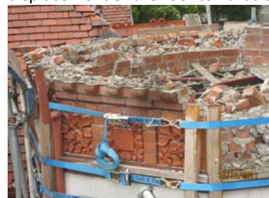
The top of the brick walls to the turret showing the corbelled brickwork to the eaves and the terracotta frieze panels to the lintels. All has been recorded and stored.
