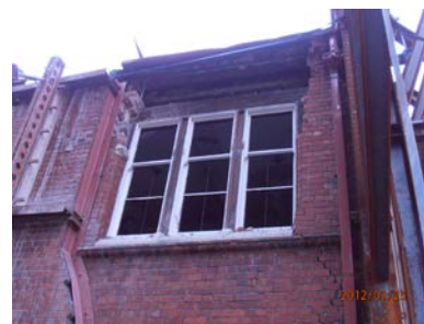
The south window of the west façade to the Council
