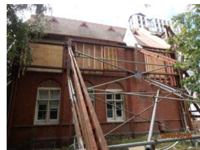
West Façade following the removal of the leadlight and stained glass windows, stone window mullions and transoms and brick to the lintols.
