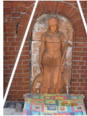
The Figurine, 'Industry', prior to removal showing the displacement of the brickwork securing the panels in place, and after removal. The damaged profiled bricks forming the alcove opening have been recorded and stored enabling the reconstruction of the figurines.
