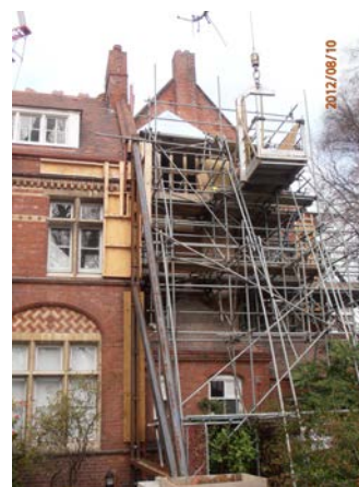
The north-west stair well partially concealed by the stabilising scaffold.
