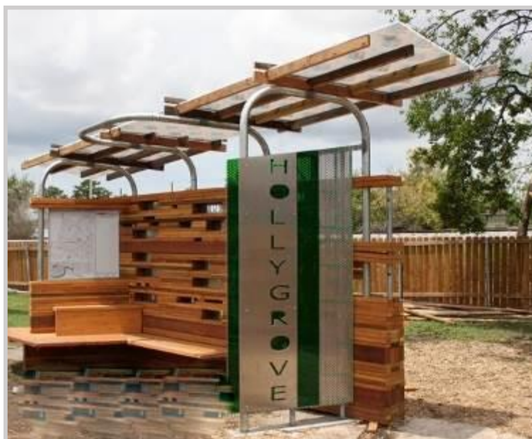
The new bus shelter created by residents with local design students and using recycled and donated materials
