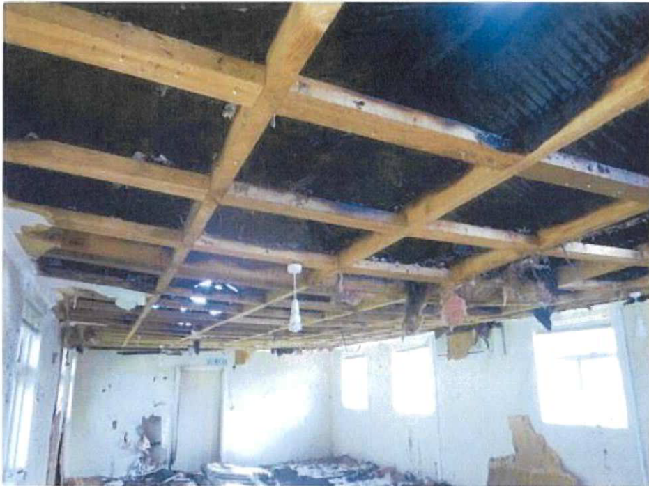
Roof trusses completely burned through causing loss of ceiling support
