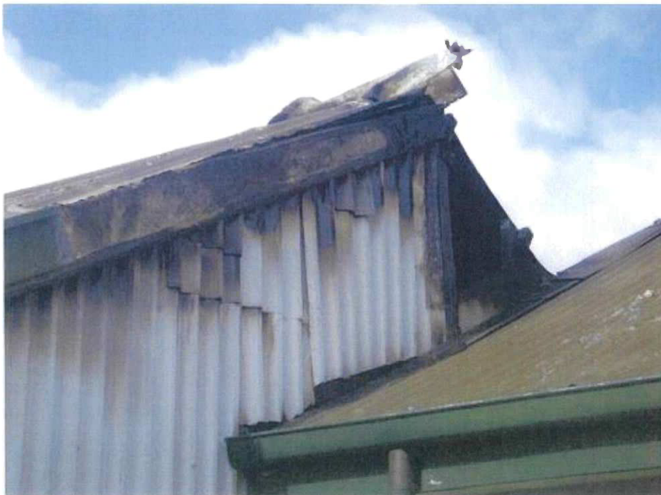
Fire passed into adjacent hall roof causing damage.
