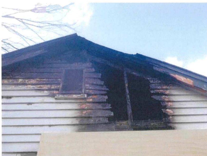
Fire entered into roof structure at this location
