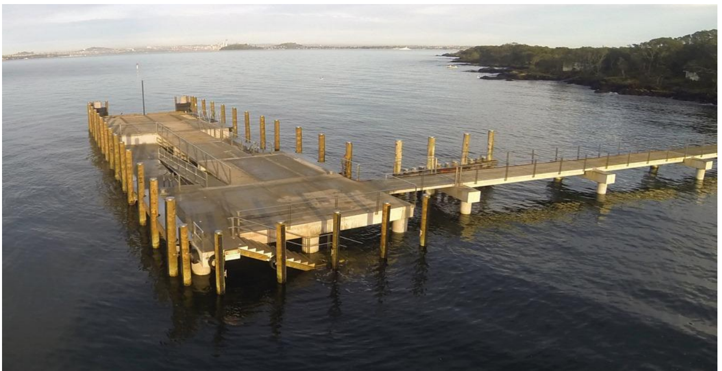
Figure 4.5 Rangitoto Island Wharf, Auckland. Example of reinforced concrete wharf
