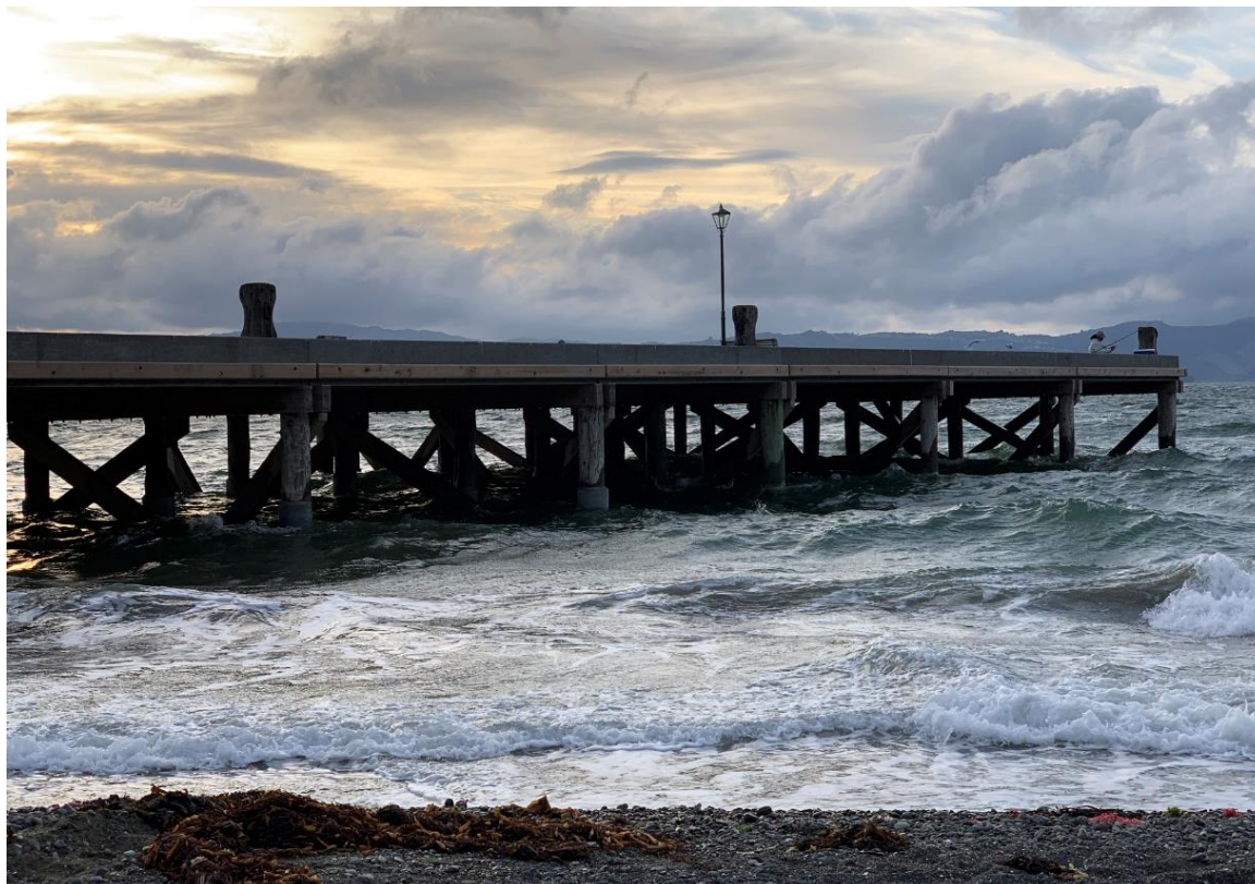
Figure 4.3 Photograph showing refurbished wharf with timber bracing, piles and walers, concrete edge beam and deck.
