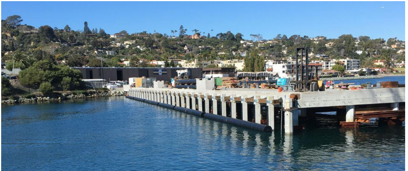
Figure 4.4 UCSD Nimitz Wharf. Example of reinforced concrete wharf
