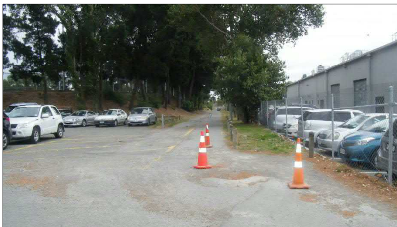
Railway underpass – southern approach.
