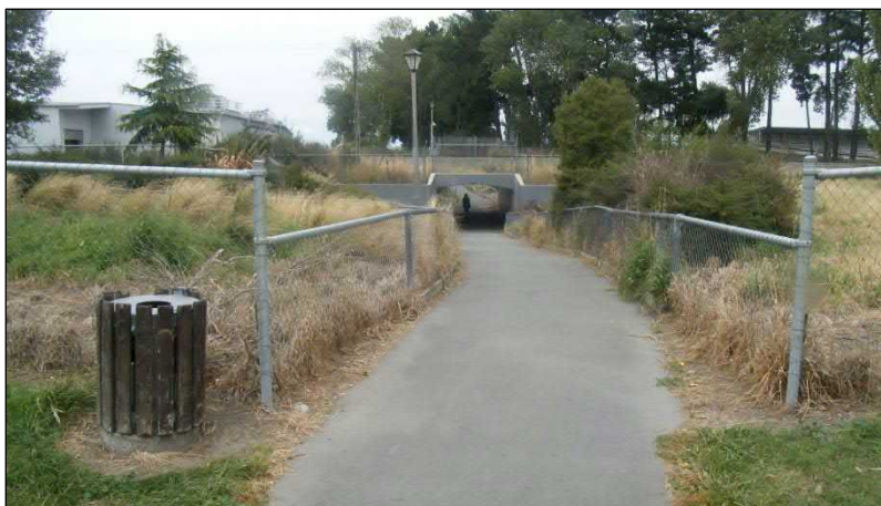
Railway underpass – northern approach.
