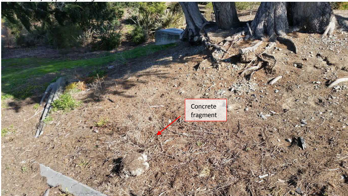
Photograph 4: A concrete fragment visible on the ground surface by the southwestern embankment. Date taken: 27/08/15; photo facing west.
