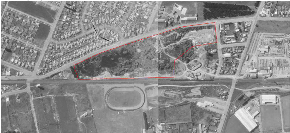
Figure D4: 1965 aerial of the site and surrounds. Red line represents the indicative site location. Source: Canterbury Maps.
