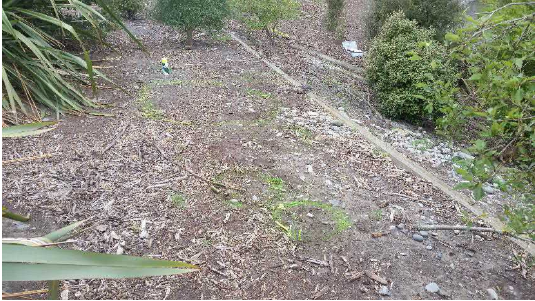
Above: Photograph 7 - top of south western embankment (Area 1)
