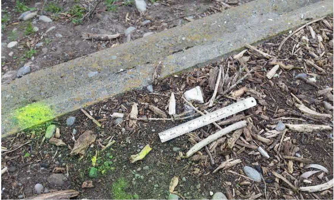
Above: Photograph 9 - example of ACM fragment, in-situ (Area 1)
