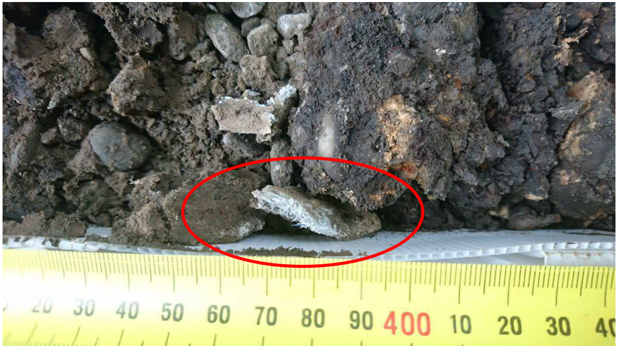
Photograph 5 – example of asbestos containing material (cement board materials) (Borehole 111 at 0.7 m bgl).
