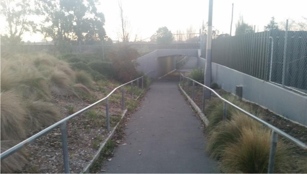
Figure 4-4: Denton Park/Kyle Park Railway Underpass
