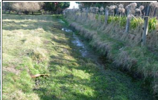
J: Tysons Drain Branch No 1 West, looking upstream.
