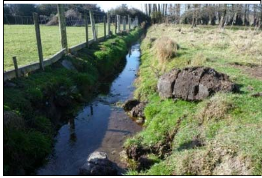
H: Tysons Drain Branch No 1 South, looking downstream.
