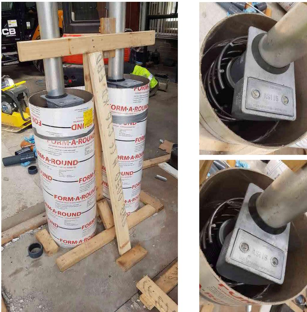
*Fig 2.2a Installation in formwork*
