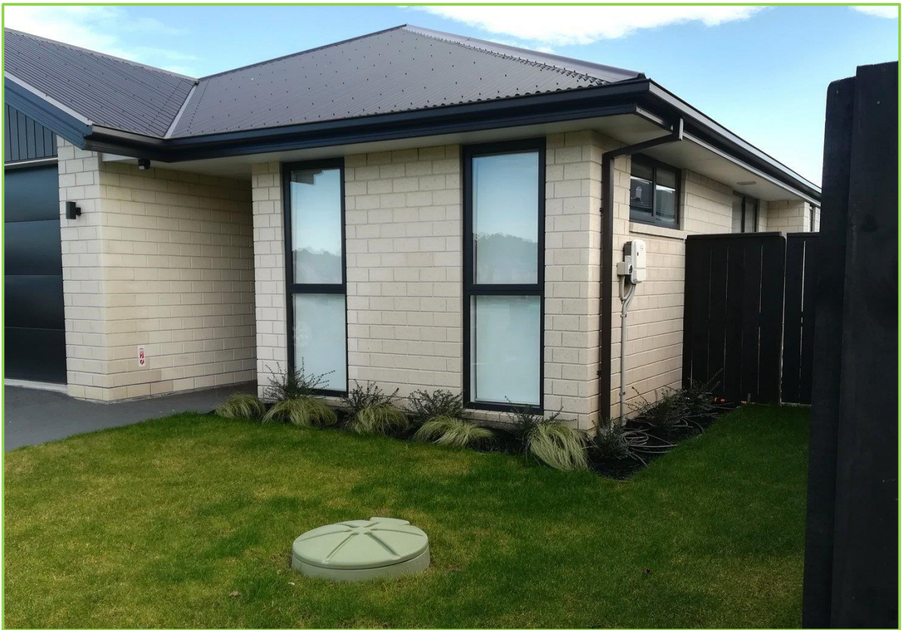
Figure 5 –Pump chamber completed installation position
