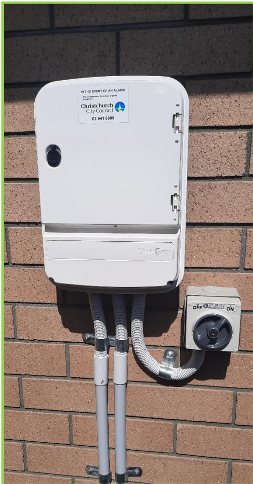
Figure 6 – Control panel completed installation position
